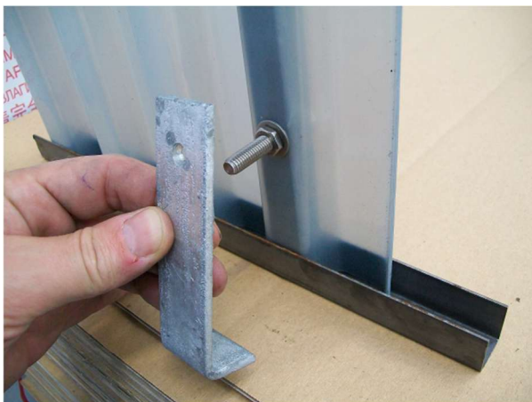
Put the fixing nut on the corner
