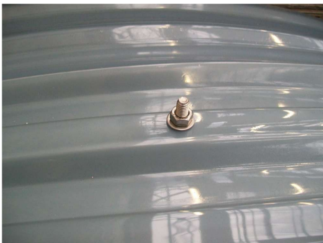
Screw the tightening bolt
