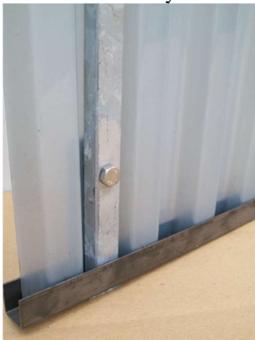
Bottom fixing details
